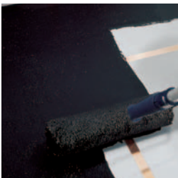
The conductive intermediate generally consists of a soot-filled, water-based epoxy resin dispersion.
