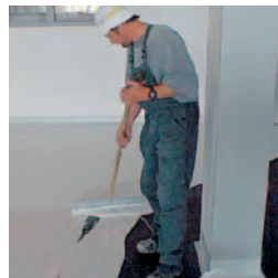
Applying the finishing coat
