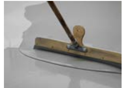
StoCrete EH 200 is applied with a squeegee ...
