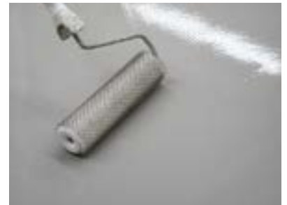
... and de-aired using a spiked roller.
