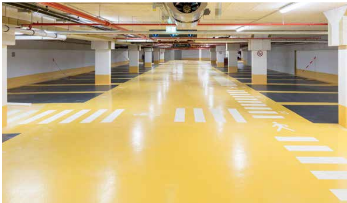
Cranachhöfe underground car park, Essen, DE Foto: Axel Hartmann
